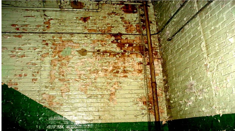
Second floor of Building #2 showing severe lead base paint. Similar examples were observed during our walk through of other buildings.
