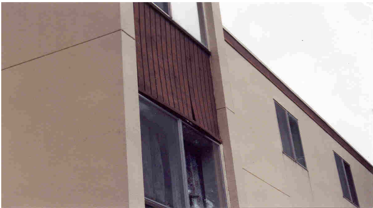
No. 2, Building A – Exterior siding panel is rotted. This condition was noted in several places.
