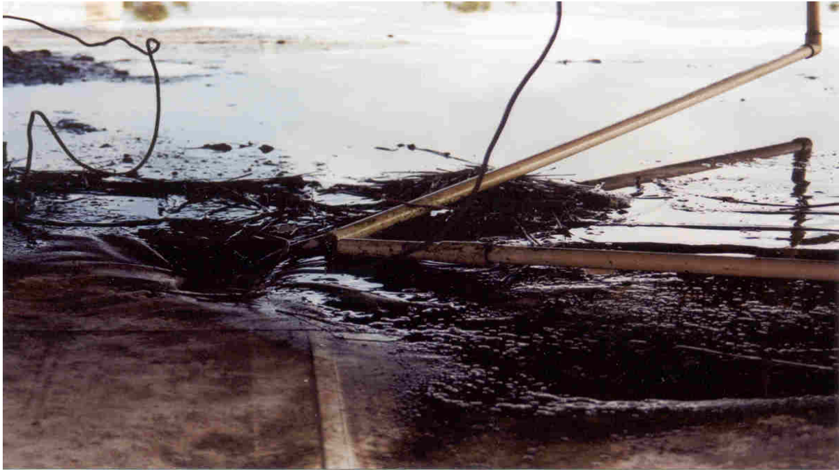
No.1, Building A Roof – Pooling water due to defects in AC condensation lines.
