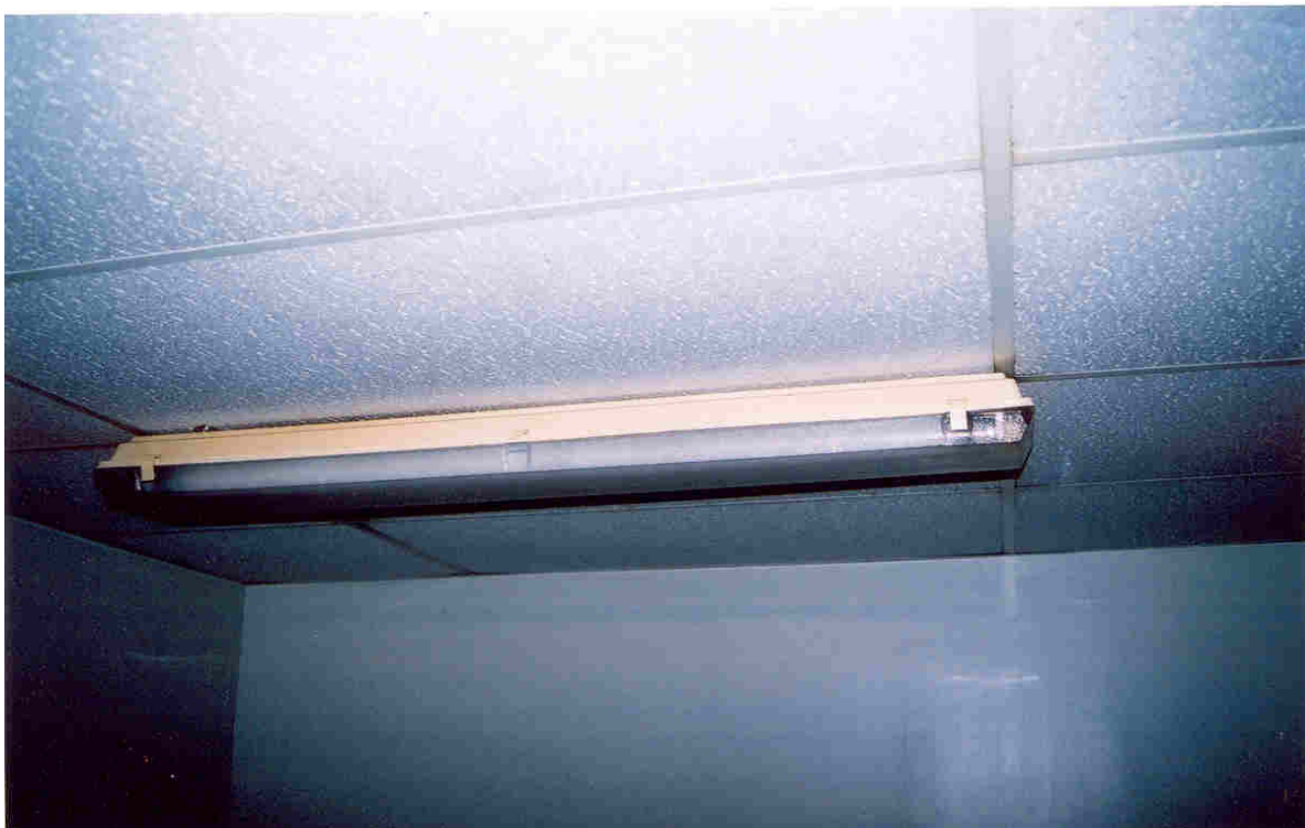
No. 5 & 6, Buildings A and B, stairwells – Burned out or missing bulbs and missing lens covers.
