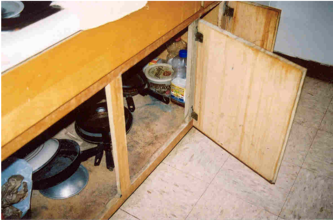
No. 21, Unit 103B – Kitchen cabinets were replaced, but staining was incomplete and shelving was omitted.
