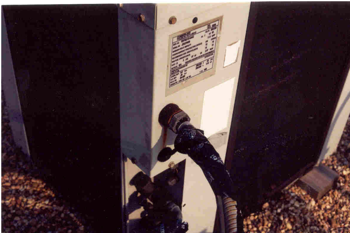
No. 10, Building B Roof – Exposed AC electrical wires due to separated cable sheathing.
