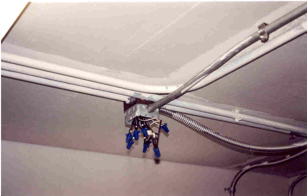
No. 8, Building A- Meter room – exposed wiring
