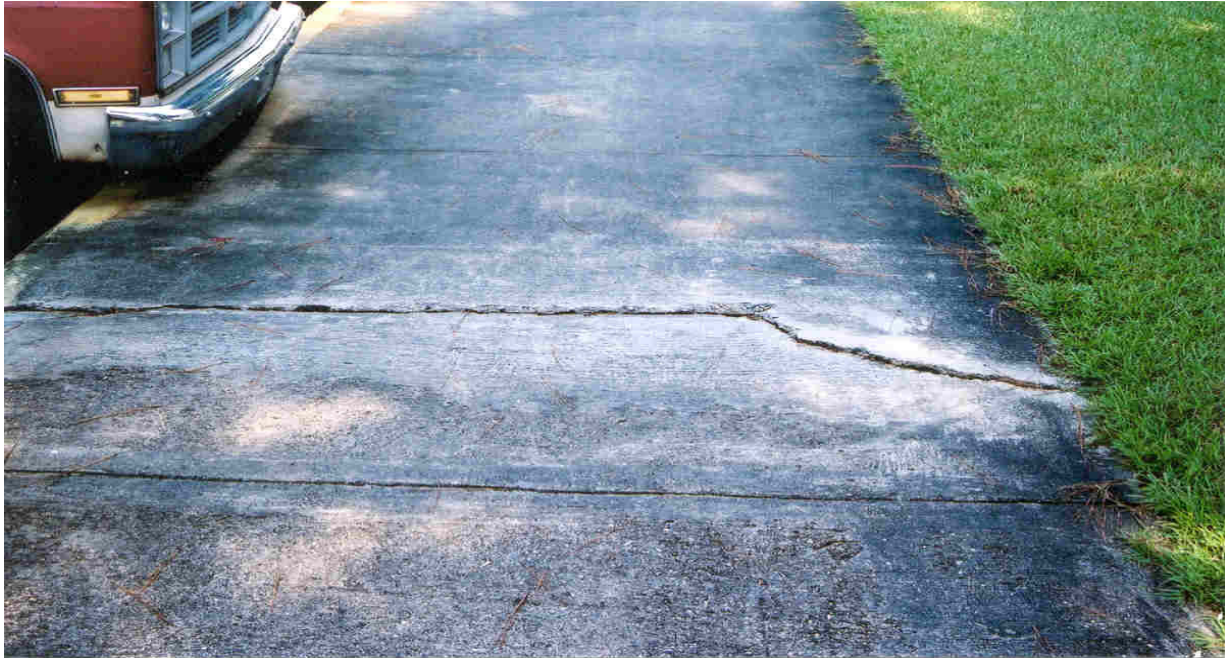
No. 3, Building A – Crack and upheaval in walkway is a tripping hazard.
