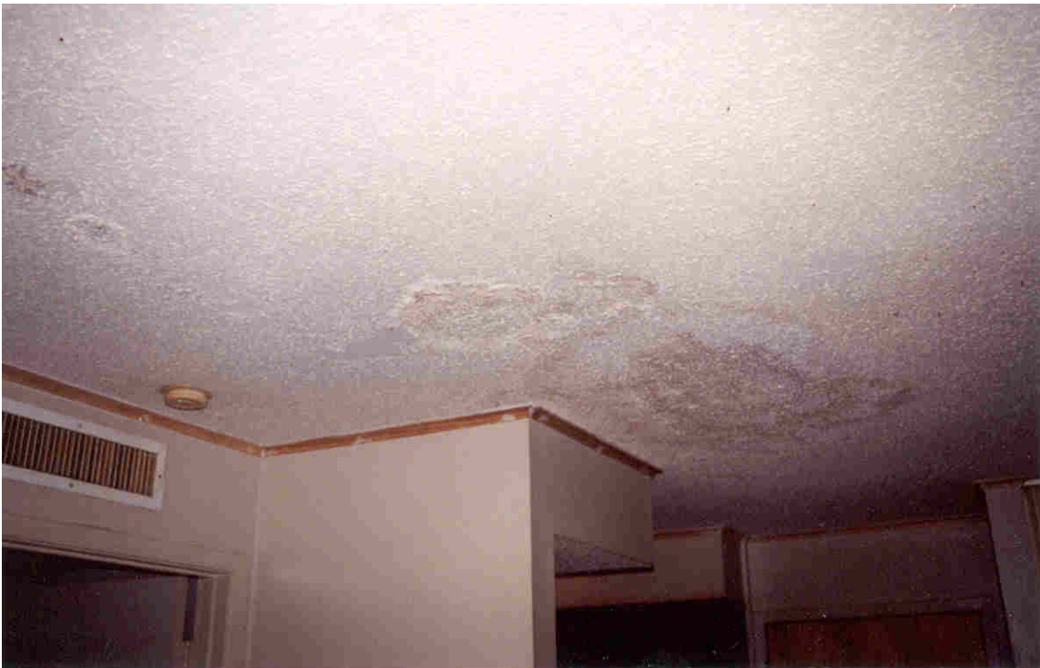
No. 28, Unit 303A – Water damage to living room ceiling has not been repaired. Trim molding was not painted.
