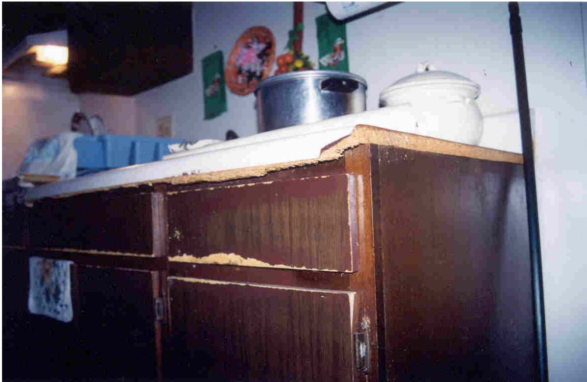
No. 17, Unit 214A – Kitchen sink cabinet is delaminating. Countertop underlay is crumbling. Similar conditions were noted in nearly all units inspected.
