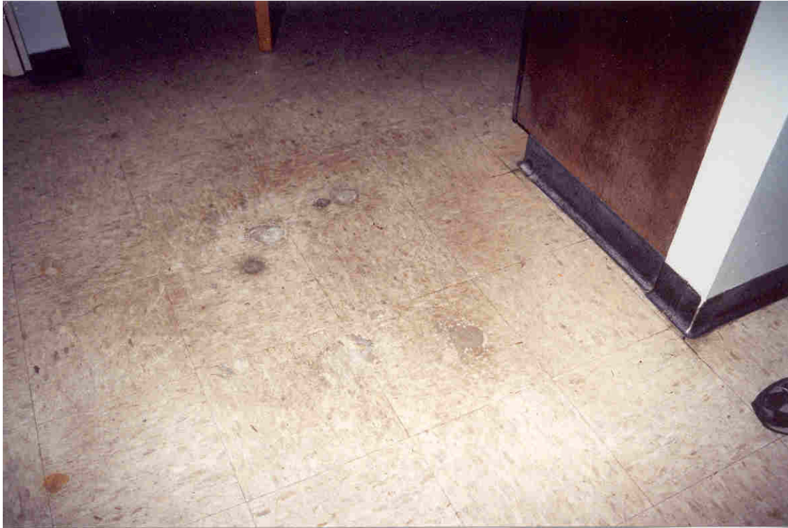
No. 25, Unit 308A – Dining area floor tiles are completely worn through.
