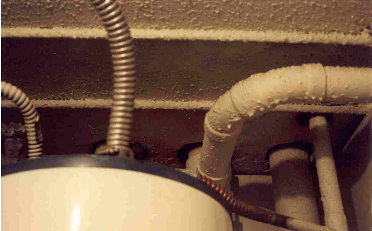
No. 7, Unit 101A – Water heater closet – plumbing holes in ceiling not sealed to provide fire barrier.
