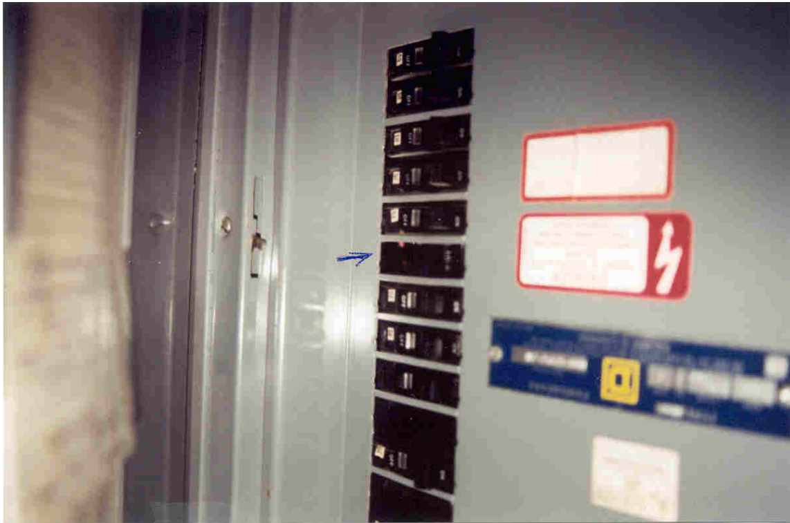
No. 9, Building A Meter room – Electrical breaker box, open breaker slot covered with tape.
