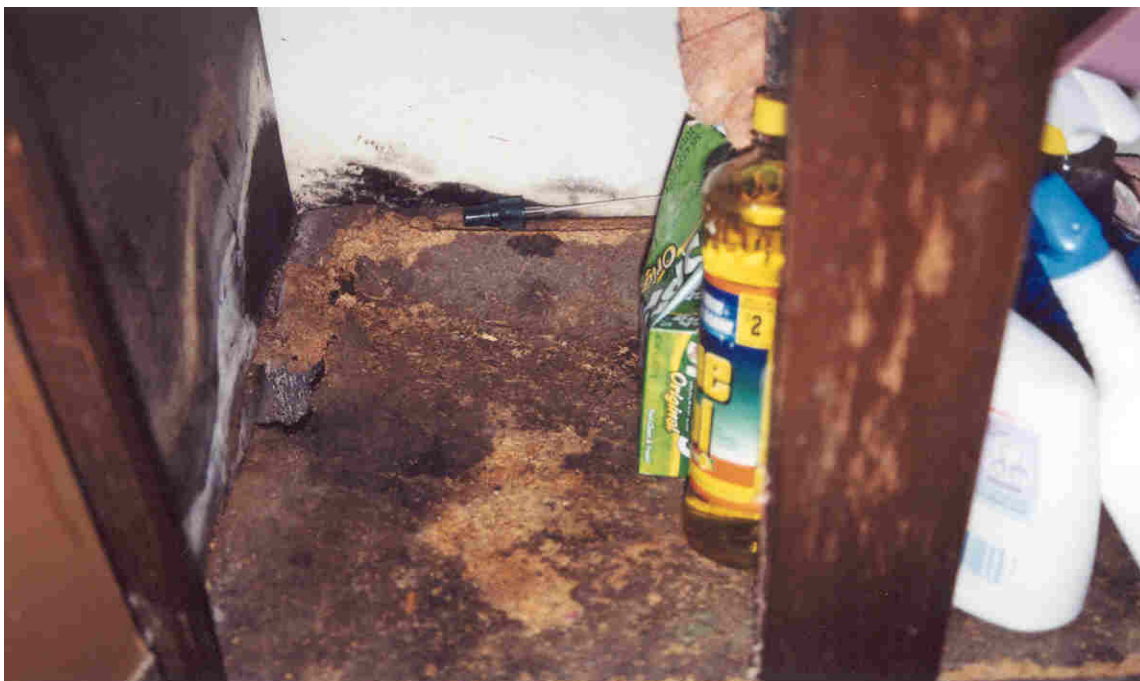
No. 18, Unit 314A – Kitchen sink cabinet, sidewall and bottom shelf are rotted out and mildewed.
