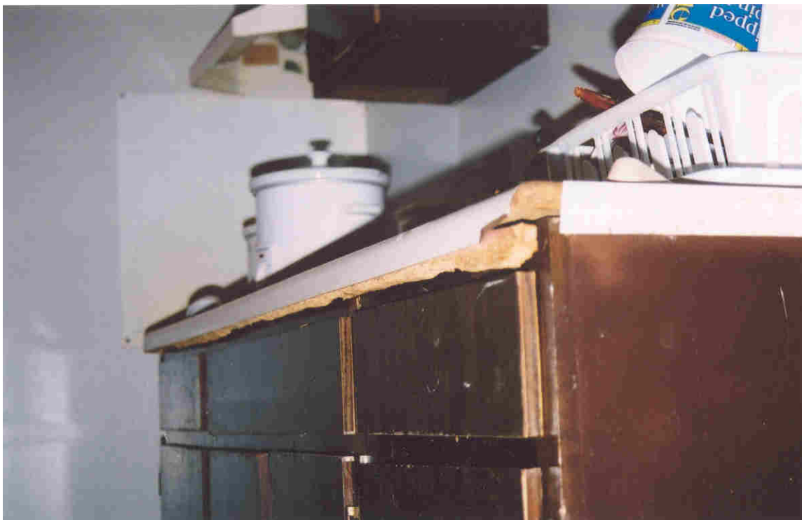
No. 14, Unit 112B – Arts and Crafts room – sink cabinet is delaminating and countertop underlay is crumbling.
