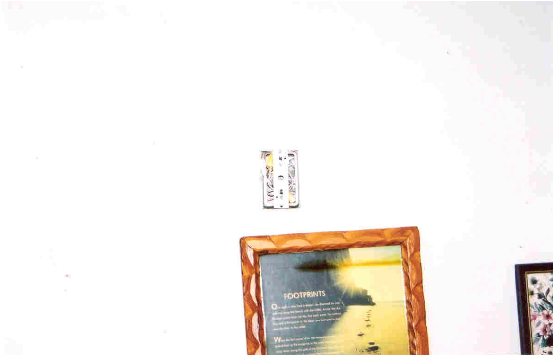
No. 15, Unit 112B – Arts and Crafts room – exposed electrical wiring.
