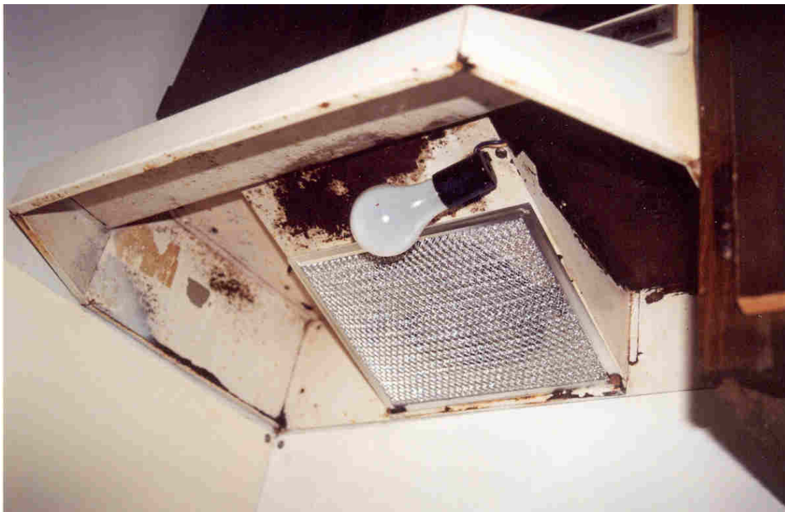
No. 16, Unit 309A – Stove vent hood is rusted, bulb cover is missing, and wiring exposed. This condition was similar in most apartment units.
