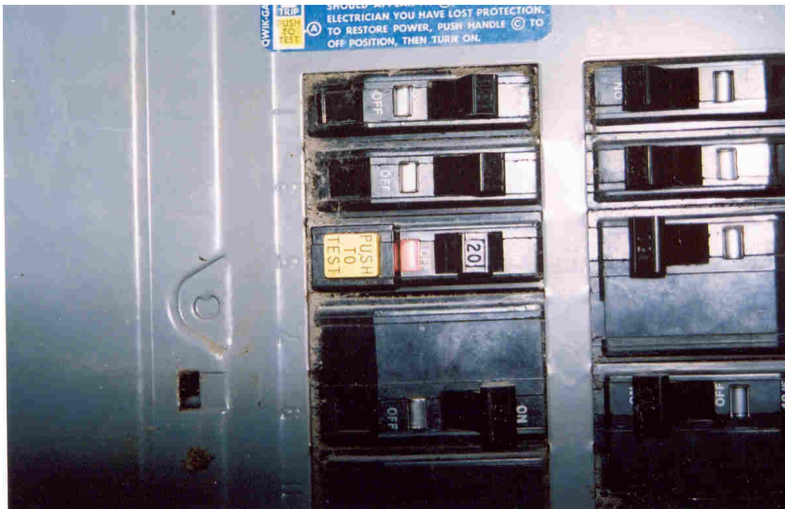
No. 12, Unit 318B – GFI breaker for bathroom was defective.
