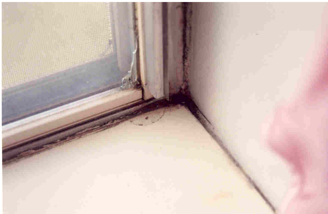
No. 29, Unit 214 A – Living room window shows deterioration and mildew due to moisture damage. The glass panes were not adequately sealed.
