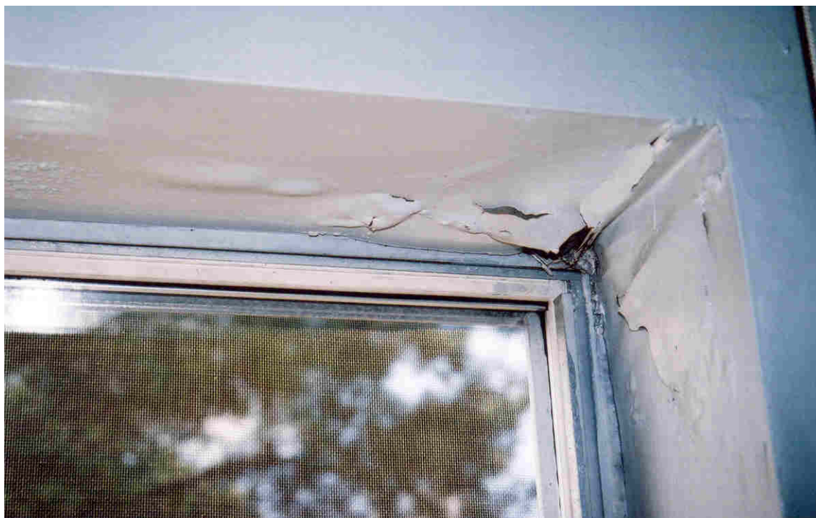
No. 30, Unit 203B – Moisture damaged drywall at window frame. The age and condition of window units makes them too difficult to operate, and subject to moisture intrusion.
