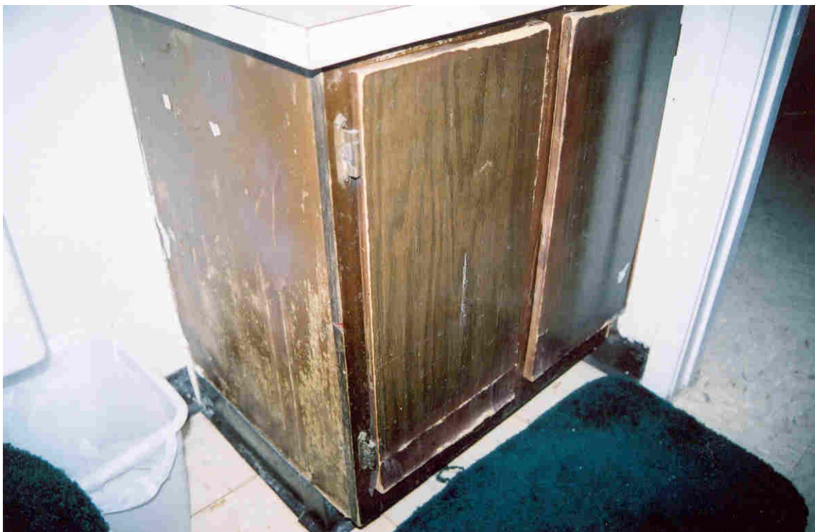
No. 22, Unit 203B – Bathroom vanity is delaminating. Side finish and inside shelf surface are deteriorated and not impervious to moisture.
