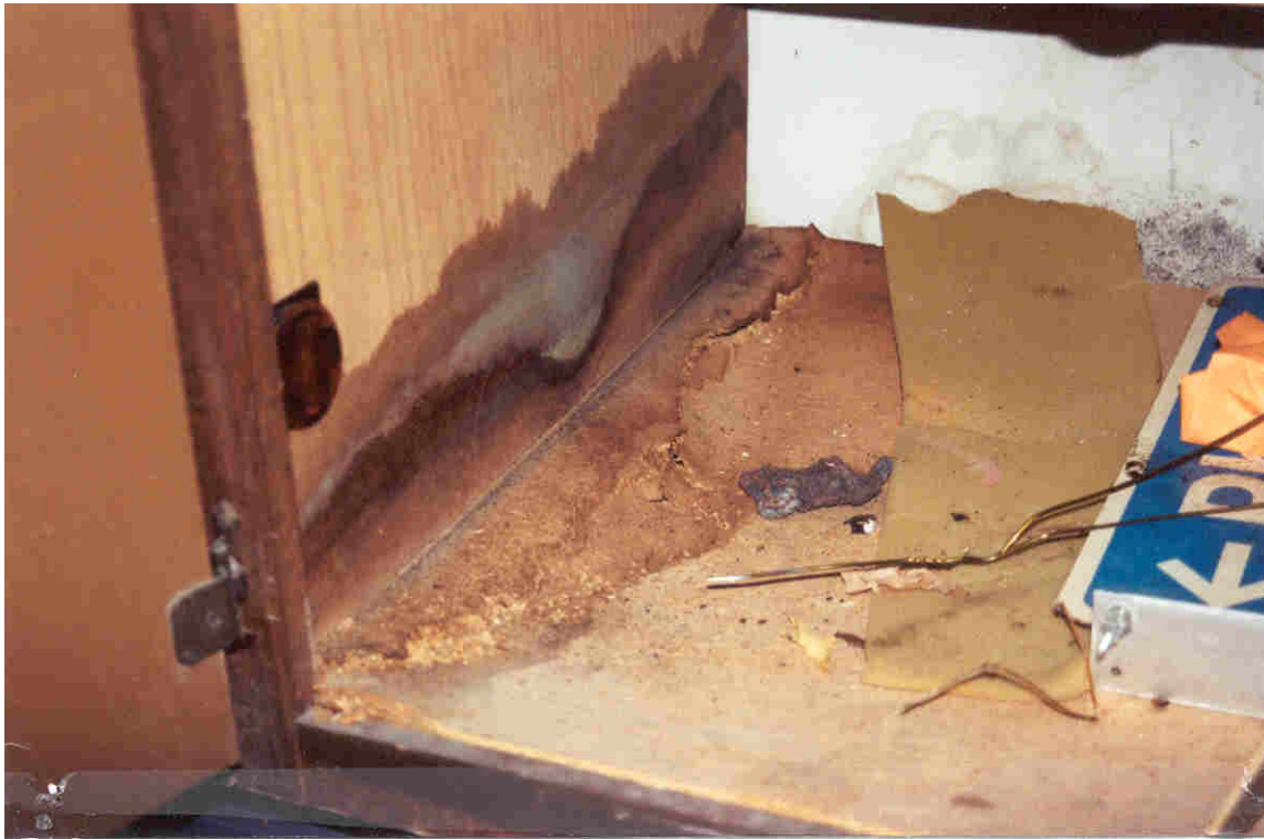
No. 13, Building A Common room – sink cabinet sides and bottom shelf are rotted out.
