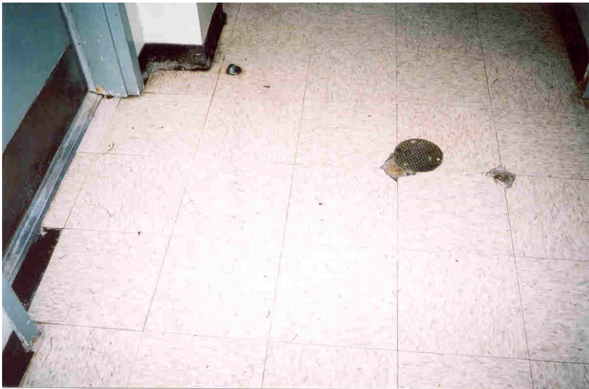
No. 24, Building B, east stairwell – missing and damaged floor tiles.
