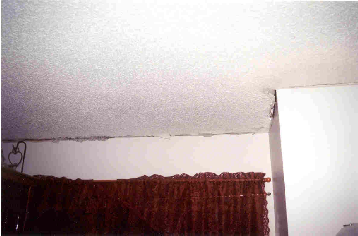
No. 27, Unit 301A – The living room ceiling to wall joint has separated.
