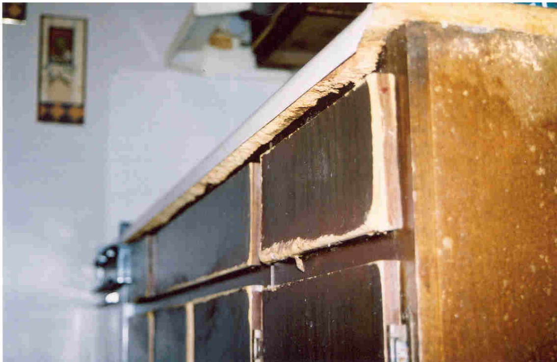
No. 20, Unit 203B – Kitchen sink cabinet has delaminated. Underlay material for doors and countertop are crumbling.
