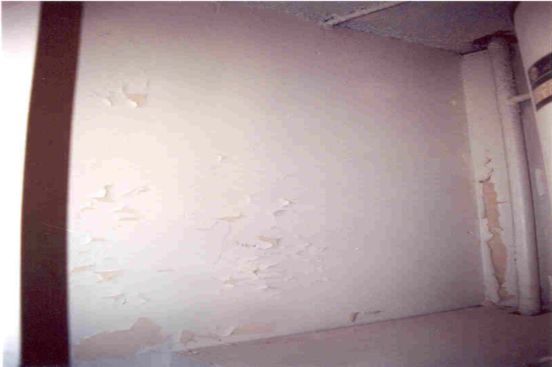
No. 26, Unit 301A – Peeling paint in utility closet. Tenant stated the apartment had not been painted in 16 years.
