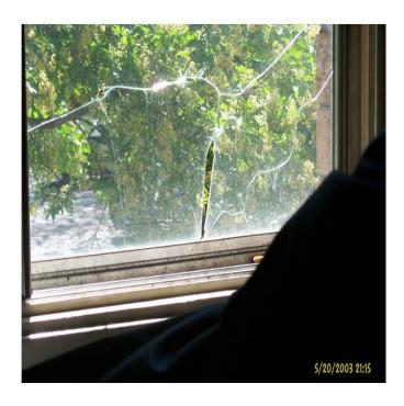
The living room window in the unit located at 1395 East Maple was missing sash ropes. The tenant used props in order to keep the window open.
