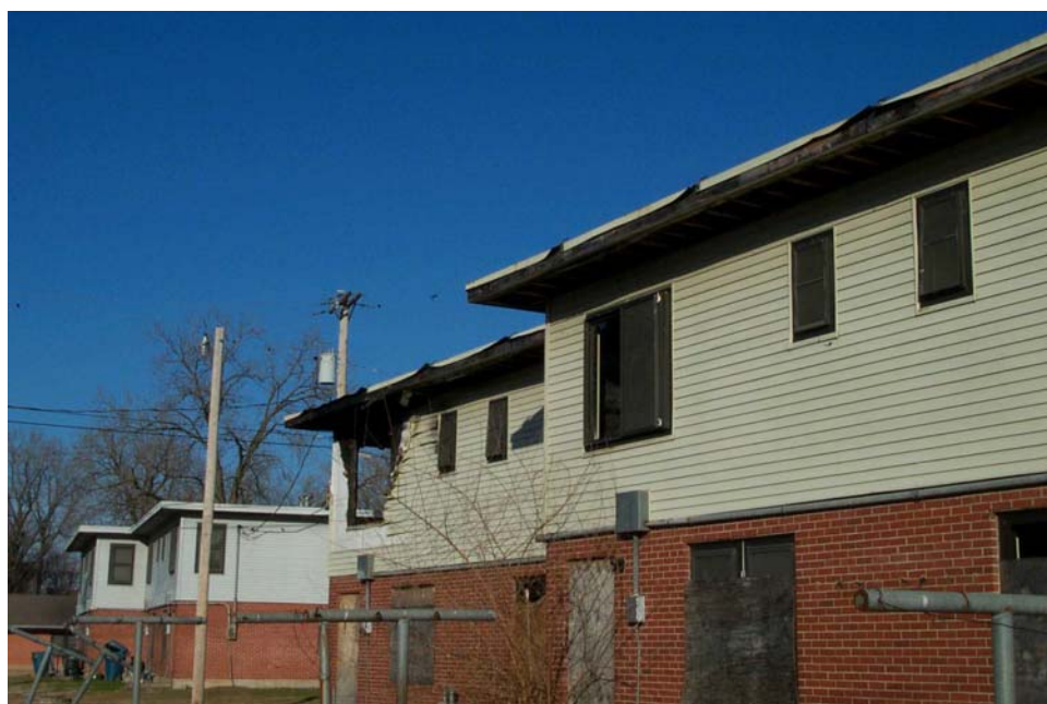
Picture 2 This picture shows fire damage at the opposite end of the same building.
