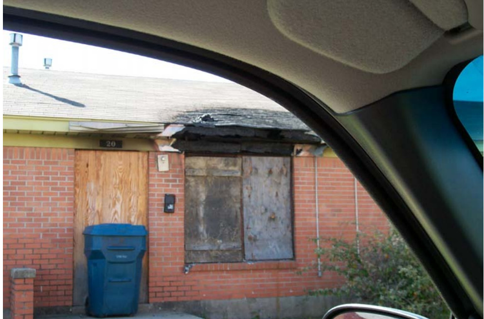
Picture 5 – Note the weathered appearance of the plywood boarding the windows.
