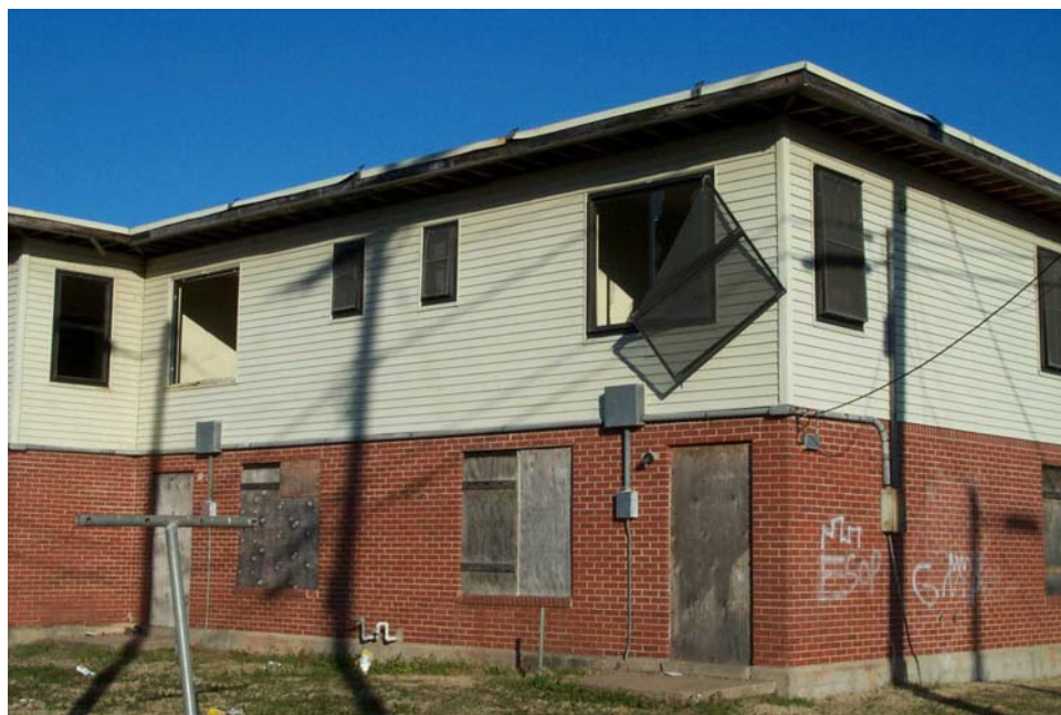
Picture 1 This building consists of four units. Note the missing windows and screen on the second floor and graffiti covered exterior.
