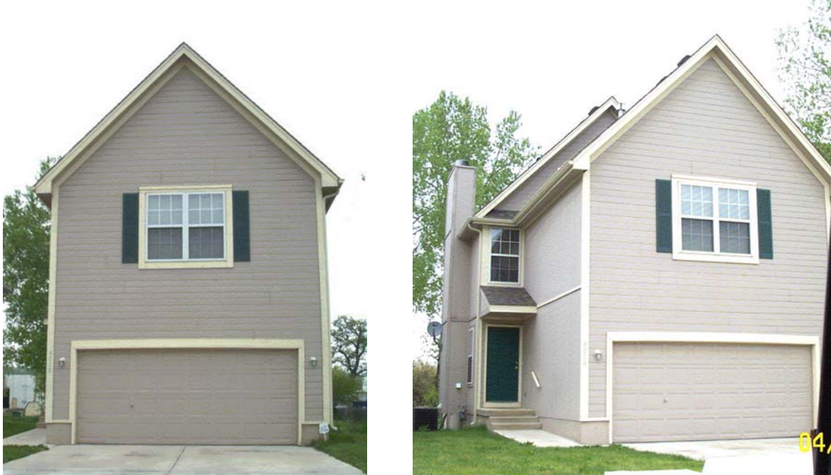
Exhibit 19. These photos show two front views of 4016 E. 16 th Terrace. This house has not yet sold although a certificate of occupancy was issued in November 2001 (4/23/04).
