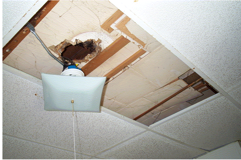
Large Hole in Ceiling and Exposed Electrical Wiring
