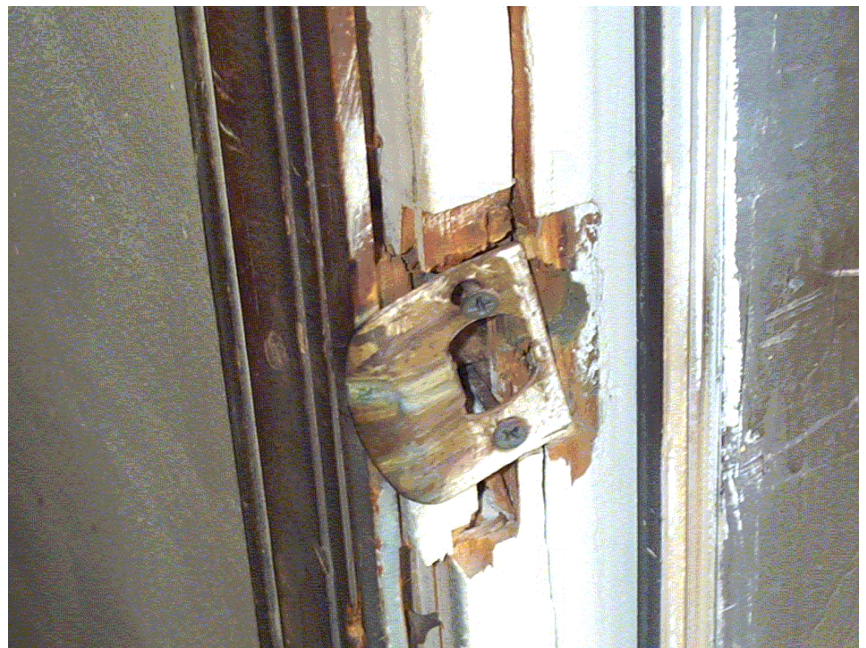
Entry Way Door Not Secure
