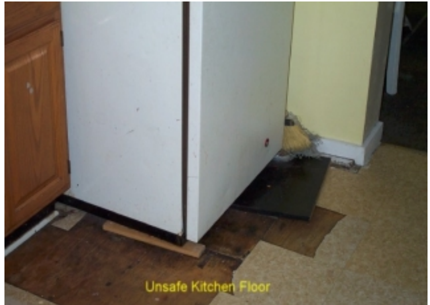
Unsafe Kitchen Floor
