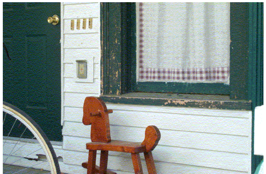
Potential Lead-Based Paint Hazard
