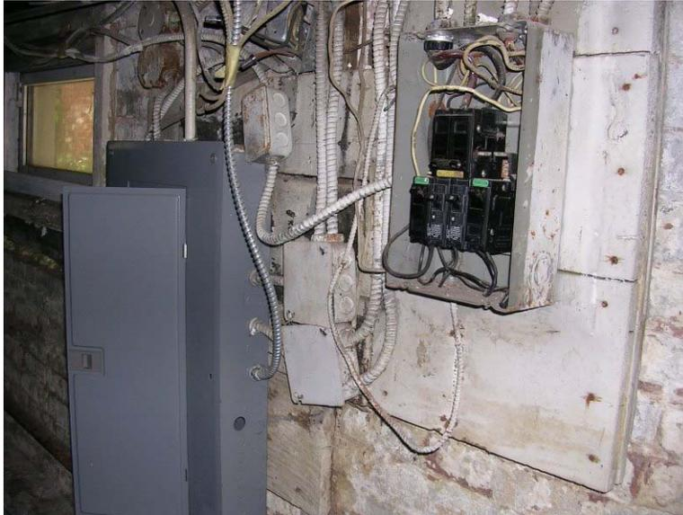
Exposed wiring on an electrical panel found during a May 5, 2006, inspection.
