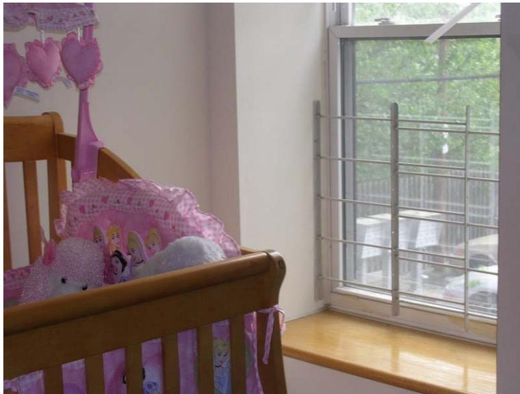
Many units contained egress deficiencies. This unit inspected on May 8, 2006 contained security bars, which could not be opened by those present at the inspection, for all windows located in this room.
