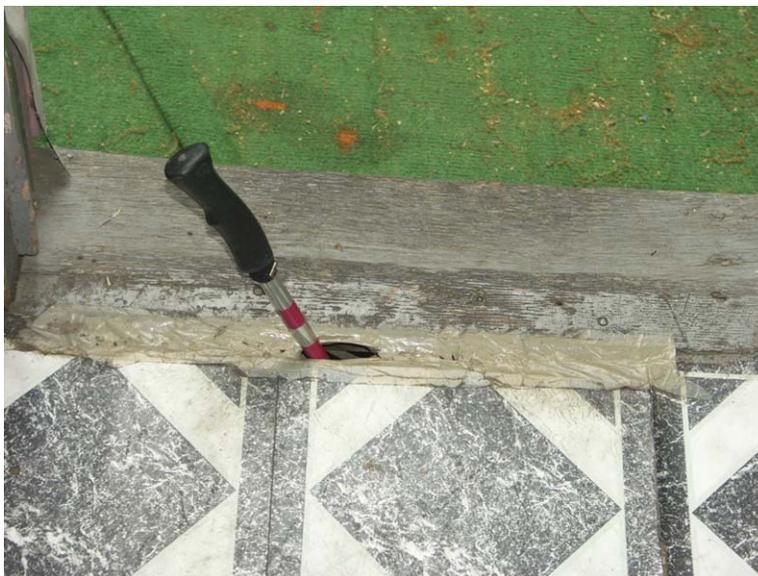
Large hole and nonconforming repair located in a kitchen
