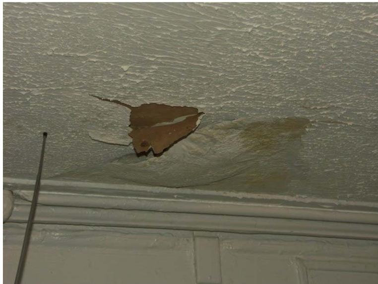
Water damage located in one unit was observed during an inspection on May 10, 2006. The leak originated from the roof above.
