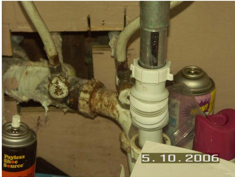
An inspection on May 10, 2006, revealed a drainage leak and nonconforming repair under a kitchen sink.
