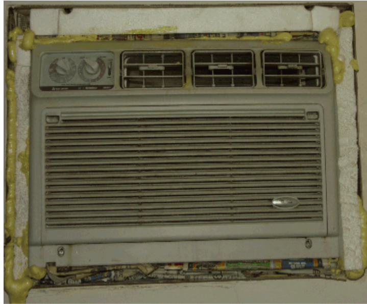
Window unit not properly sealed
