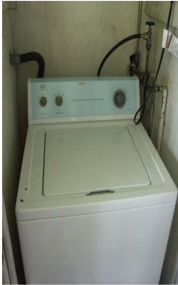
Washer not properly connected to a sewer line; water drained to backyard
