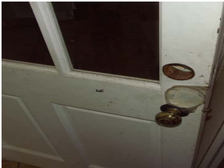
Exterior door missing door lock
