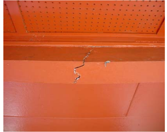
Second cracked carport beam
