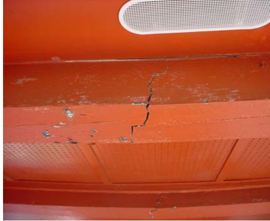
First cracked carport beam
