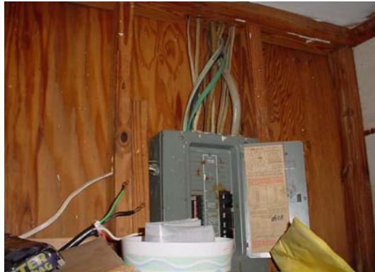
Exposed breaker box wires
