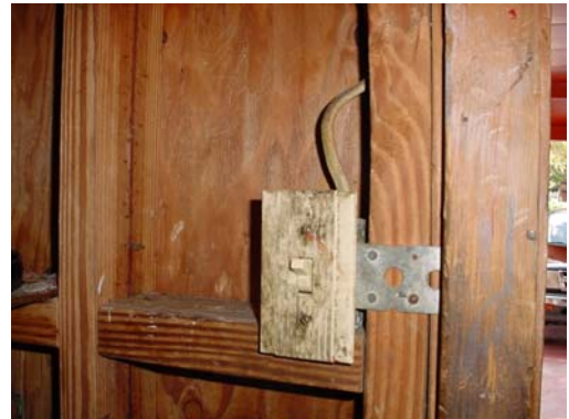
Exposed light switch wire
