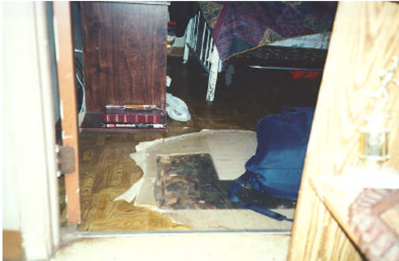
Badly deteriorated floor covering in unit 325B Liberty Street - a tripping hazard.
