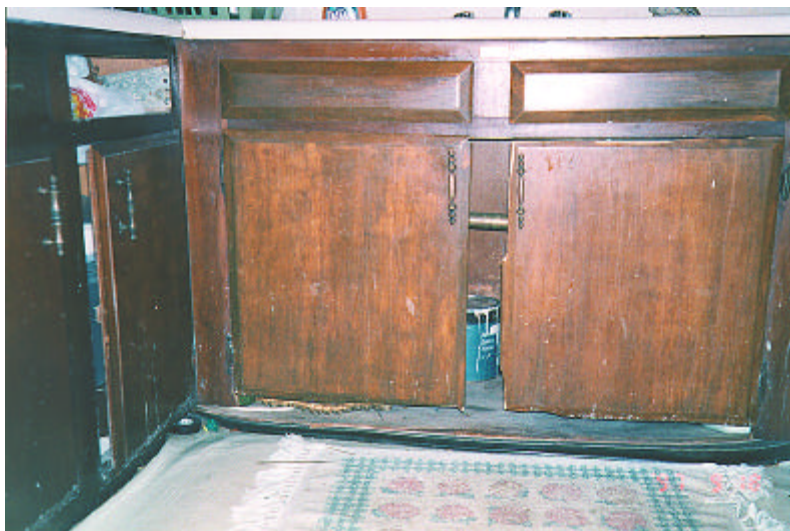
Badly deteriorated floor covering in unit 325B Liberty Street - a tripping hazard.
