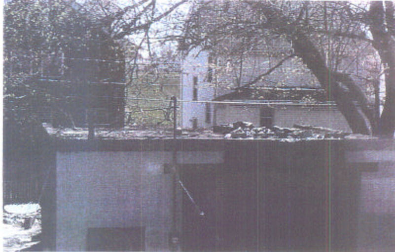
FHA Case 372-2618957. The specification for rehabilitation work items required new roofing which was not installed.
