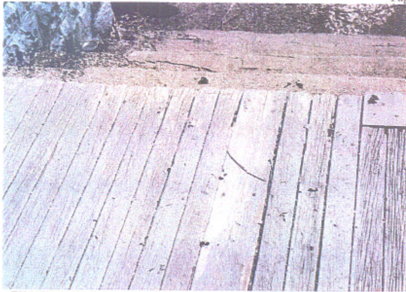
FHA Case 372-2647057. The specification for rehabilitation work items required 798 square feet to paint porch ceilings and deck at $1,185. The work was not done in a professional workmanlike manner.
