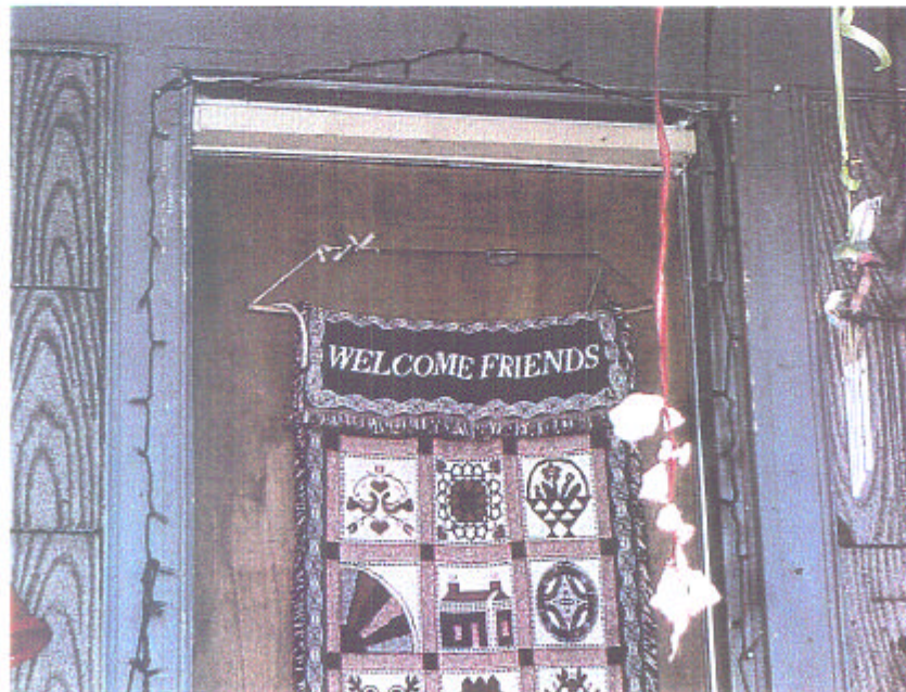
FHA Case 372-2618957. The exterior door was installed for $364. But, the door did not fit the span. So, the contractor placed a 2X4 below the header without insulating and trimming the new header. This created an aesthetically inferior product not to mention a security risk.
