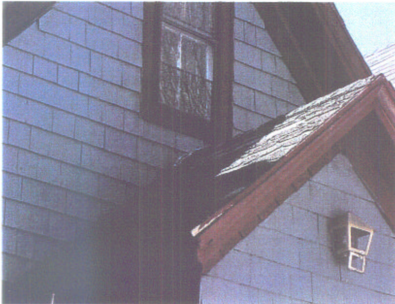
FHA Case 372-2655733. The specification for rehabilitation work items required new roofing throughout entire house for $4,000. We found portions of the roof that were not completed.
