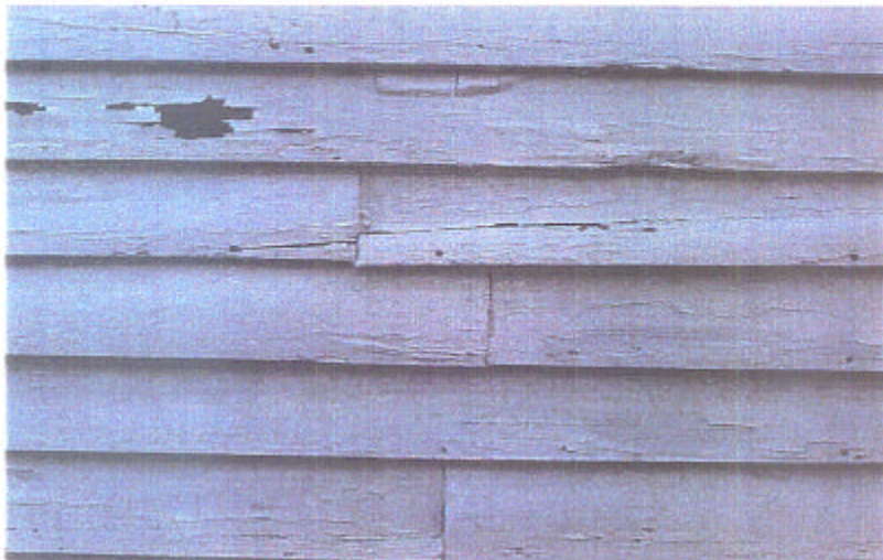
FHA Case 372-2644260. The specification for rehabilitation work items required the contractor to scrape, sand smooth, and paint a minimum 2 coats of good quality paint at a lump sum amount of $3,420
