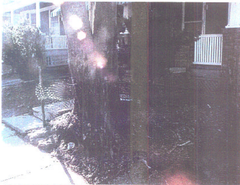
FHA Case 372-2594476. The specification for rehabilitation work items required the removal of an existing front fence. The work item was not completed.
