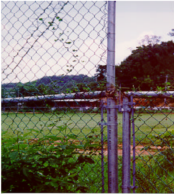
Parcelas Nuevas Baseball Park Fence welds were not properly treated. Grantee inspector indicated that the fence will soon collapse because of the rust.
