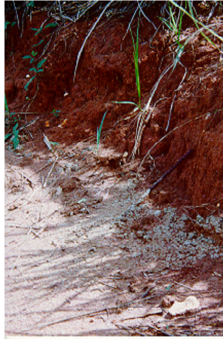
Sabana Hoyos Storm Sewer System Concrete not properly spread
