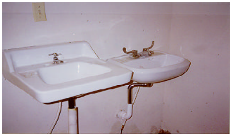
Los Caños Bathroom Facilities Improperly installed sinks in the bathroom (not handicapped accessible). Park neighbors completed plumbing.
