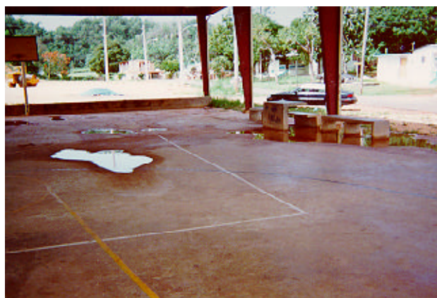
Parcelas Bithorn Basketball Court -Construction debris not cleared and court floor not properly leveled causing water to stand on the court
