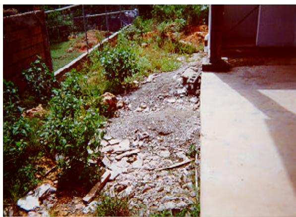
Parcelas Bithorn Basketball Court -Construction debris not cleared and court floor not properly leveled causing water to stand on the court
