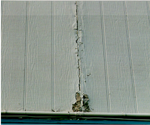
Building 20 - The siding is rotted and shows a lack of caulking.
