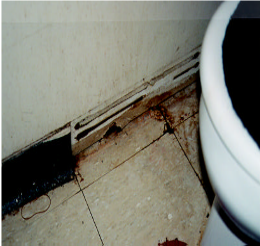
Unit 74 - The trim and floor near the commode were damaged.
