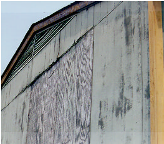
Building 50 - The siding is starting to rot and the trim is not painted.
