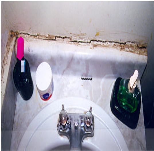
Unit 42 - The counter top on the bathroom vanity was separating from the wall.
