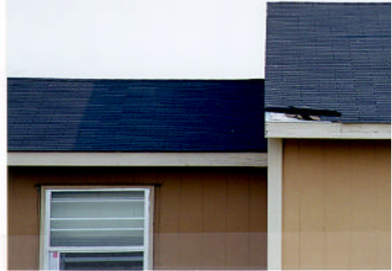
Building 60 - New roofing was installed over deteriorated decking and is coming loose.
