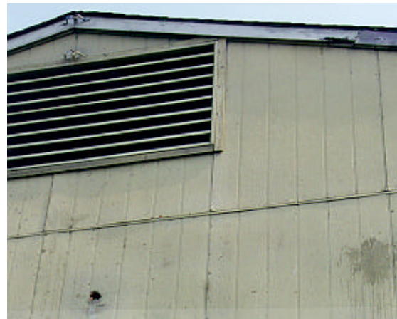
Building 70 - The siding and trim are starting to rot. There is also a hole in the siding.
