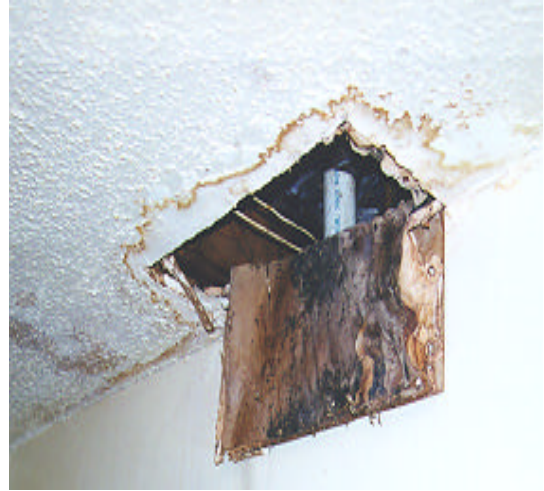
Unit 51 - The kitchen ceiling was damaged by leaking water.
