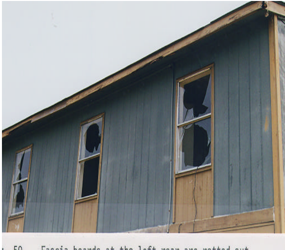
Building 50 - The trim is rotted, and hazardous broken glass is still in the window frame.
