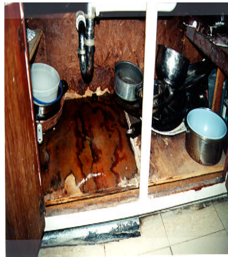
Unit 41 - The kitchen cabinet was deteriorated with signs of water damage.
