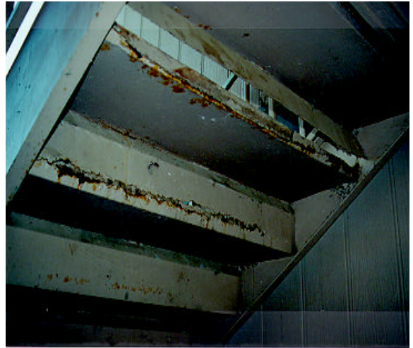
Building 30 - The stair pans are rusted out.
