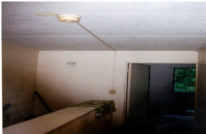
2215 Janie Poe - The smoke detector was not properly wired. The smoke detector was wired to an electric switch that could be turned off by the switch. Also, there was no smoke detector on the first floor; only one smoke alarm was on the second floor of the two story unit.
