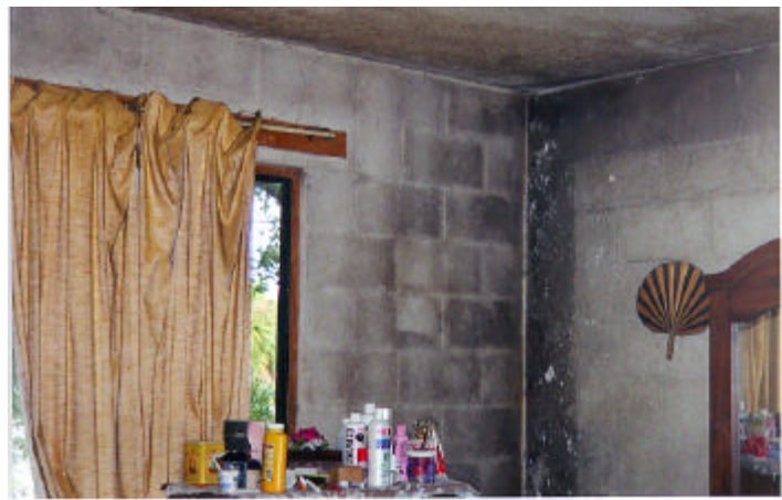
2508 Janie Poe - Mold on bedroom ceiling and walls.
