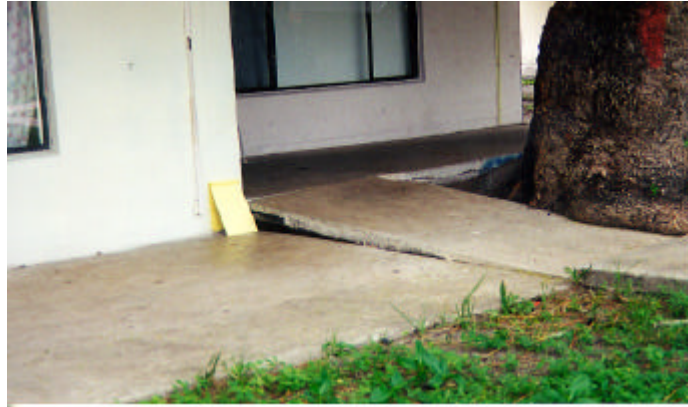
2252 Janie Poe - The tree had caused damage to the sidewalk, porch, and foundation.
