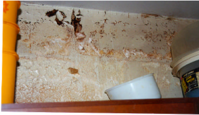
2548 Janie Poe - The wall above the kitchen cabinet was moldy and the paint was peeling.
