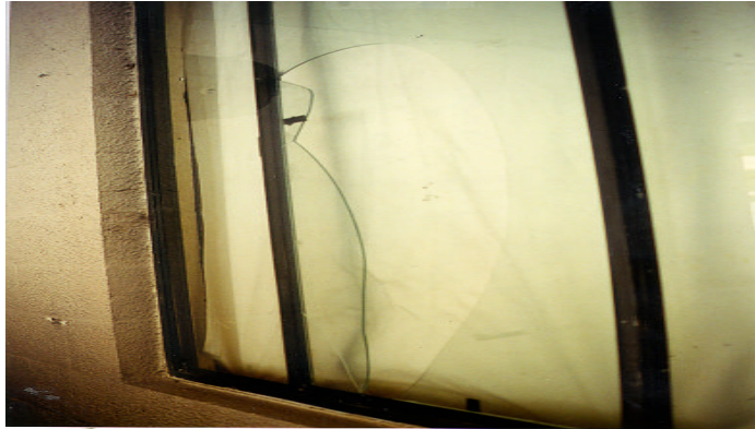
2415 Janie Poe - The living room window was broken, leaving a large hole with sharp edges.
