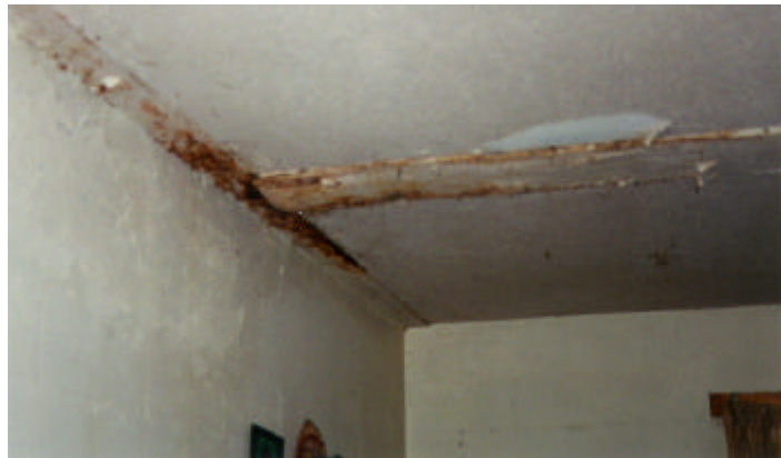
2415 Janie Poe - The living room ceiling was damaged from leaks in the upstairs bathroom or soil pipe running through the living room ceiling.
