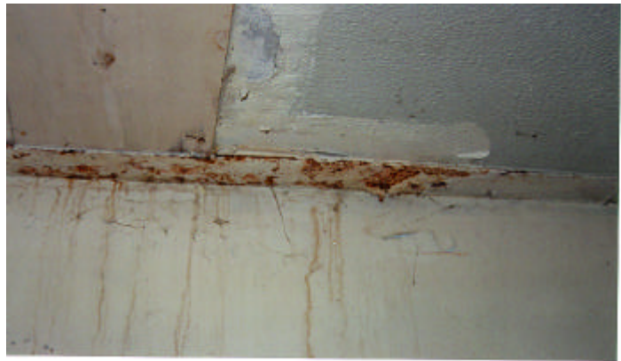
2 508 Janie Poe - The living room ceiling and walls were damaged from leaks in the upstairs bathroom.
