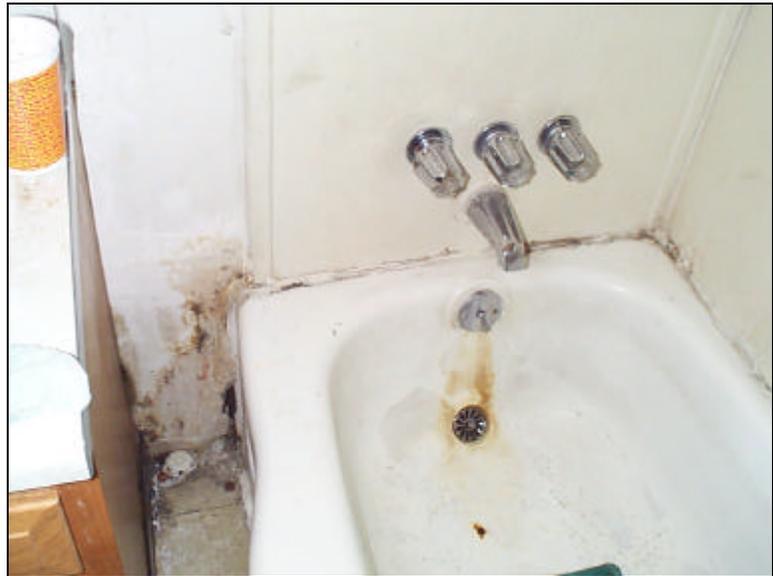
The apartment at 2521 East 33<sup>rd</sup> Street for Longwood had damaged drywall and the bathtub caulking needed to be replaced.
