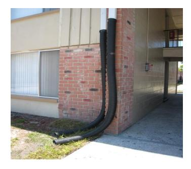
PVC piping will be allowed provided it is properly installed (as shown in the photo below) and is painted to match the adjoining gutter/downspout system.
