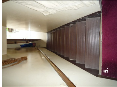
Photos 5, 6 and 7 - Unit interiors at McIntosh Homes, which may have been considered appropriate in 1952, are extremely inadequate by today's standards. Access stairs in second story units do not meet standard building code requirements and are constructed of wood with closed risers, damaged wood treads and missing handrails which represent a safety hazard for residents. All units have inadequate room sizes with only one bathroom and small combined kitchen and dining area - and inadequate layout of kitchen spaces - lacking counter space in key locations. Bedroom sizes are extremely small - with some of the bedrooms lacking circulation space once furnished.
