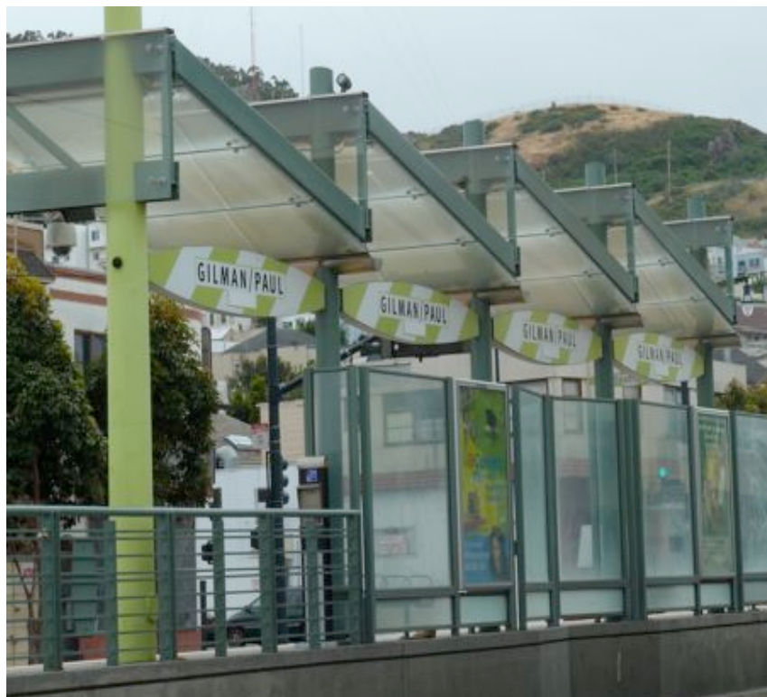
T-Third Station at 3 rd Street and Gilman Avenue.
